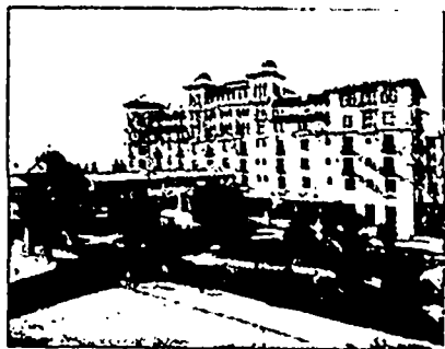
An Absolutely Fireproof Building Completed in 1898.
