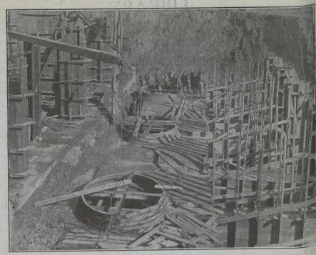
Showing Draft Tube from Wheel Chamber, Welland Pumping Station.
