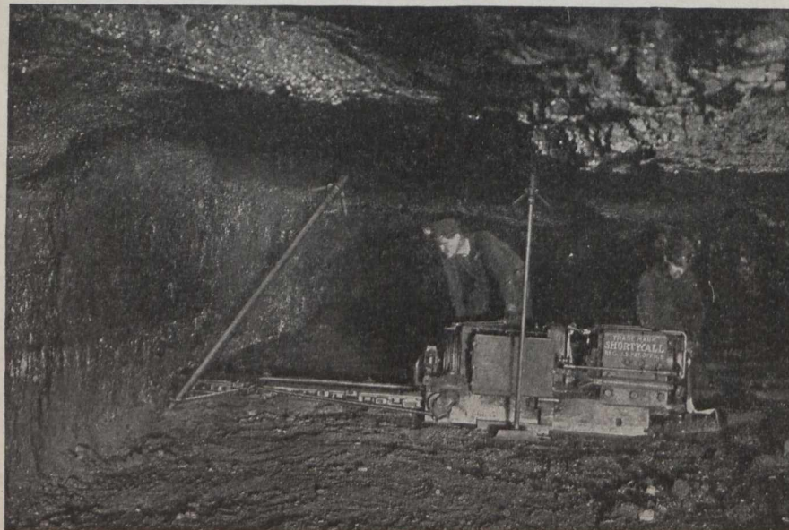
Figure 2. Illustrating method of sumping
