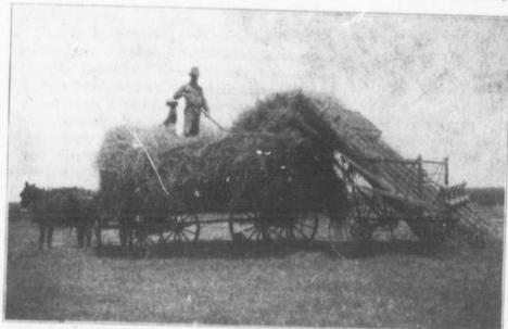
Hay Loaders Figure Largely in the Work of Present Day Hay Making
