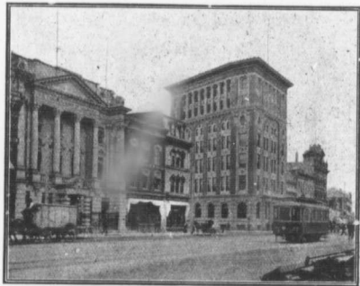
SOME FINE BANK BUILDINGS IN WINNIPEG
