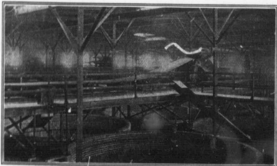
UPPER STORY OF A GRAIN ELEVATOR. (Interior)
