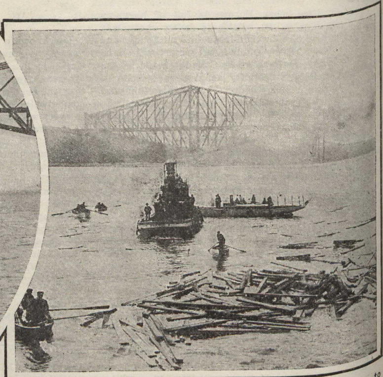
Blind, grim gravity had joined hands with some mysterious chance to upset all the calculations of engineers, the hopes of a multitude and the triumph of a nation. The great span toppled broadside. In almost the wink of an eye, free from all restraint above, rid of the pontoons that had buoyed her up, she plunged from her height twenty-five feet into the river with a vast indescribable gurgle. For a moment white foam played over the steel. And planks from the platforms above came in heaps of debris down the river.
