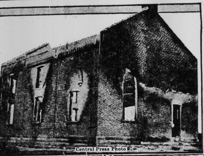
These four bleak walls are all that remain of the home of Mr. and Mrs. John B. Dennison, near Birmingham, O., after a fire in which their two children, Myra, two, and Brian, four, perished before the gaze of their frantic mother. Mrs. Dennison was working in the yard when one of the children poured oil into a basket and started the fire.
