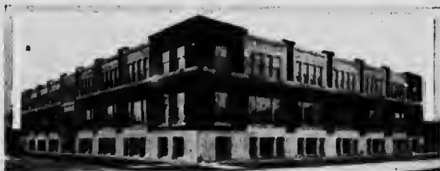
Printing Plant of The Nor'-West Farmer in Winnipeg
