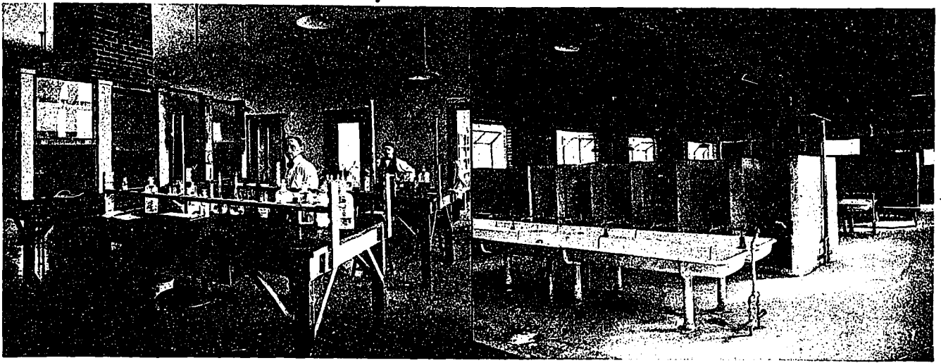
CHEMICAL OR ASSAY LABORATORY. INTERNATIONAL NICKEL COMPANY'S PLANT, PORT COLBORNE, ONT.
