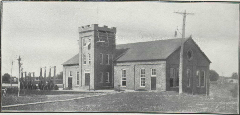
CORNWALL CANAL—POWER HOUSE, SHEIK'S ISLAND, LOWER DAM Here is generated all the electricity used to operate and light the canal
