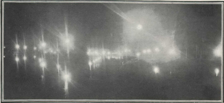
CORNWALL—LOCK 18 AT NIGHT
