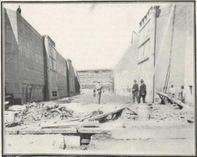
CORNWALL—LOCK 15, UNWATERED FOR REPAIRING BOTTOM
