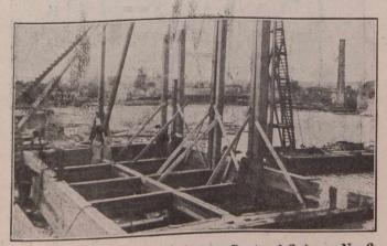
Fig. 2.-Lower Course and Binder Posts of Caisson No.2.
