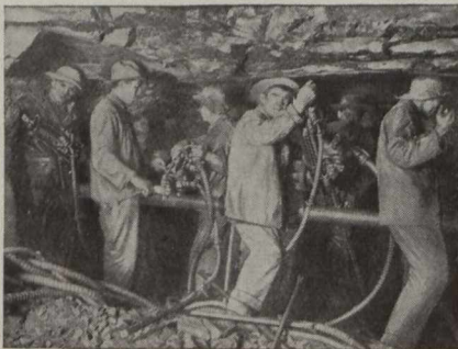
Sullivan Liteweight Water Drills in the Mt. Royal Tunnel, Montreal
