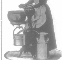
No. 6 Wingold Separator, capacity 500 to 550 lbs, per our The Wingold has all of the latest Improvements, such as split wing disk bowl, which is the fastest and closest skimming device made. Phosphor bronze bearings; low-down supply tank cut gears. Every piece and part made up of the best materials in the latest and most approved manner. Prices will be higher during 1911. Owing to increased cost of raw
