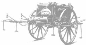
shown here, will rid an acre of potatoes of blight and bugs in 20 minutes. The only aid required is a horse. What do you think of that? Has non-clogging nozzles, 12-gallon air tank. 125 lbs. pressure guaranteed with 12 nozzles open. Agitator, clean-out and pressure relief into tank, and nozzle protector, controlled from seat. Can be fitted for orchard, vine-
