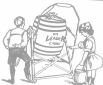
Bicycle Ball-bearings and rigid stand make the "LEADER" easy running—and there is nothing to interfere with pail being placed beneath bar to drain off the butter-milk.
