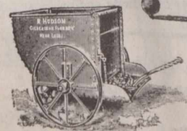
4—Furnace Coal Wagon
