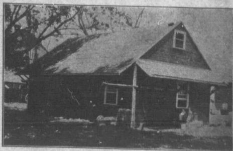
The combined milk and ice house is well equipped for city milk shipping.
