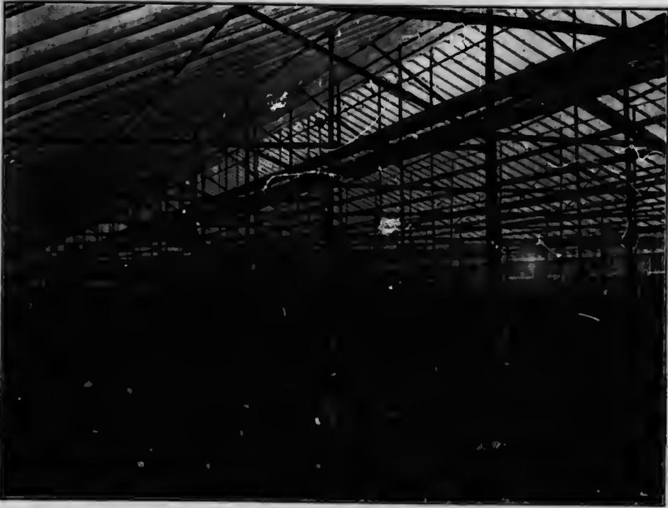
Pipe frame construction, showing the network of pipes necessary to insure safety.
