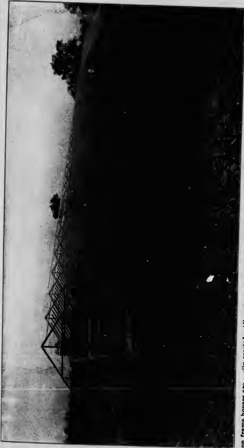
Iron frame houses are built on concrete first and then the iron rafters are raised to position. This view shows house in various stages of erection. The eave supports are set in con-
