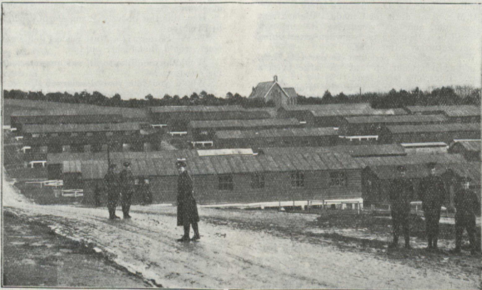
No. 1 Lines, looking East.
