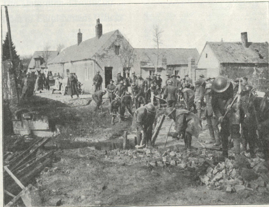
The Engineers road-making, following the advance.
