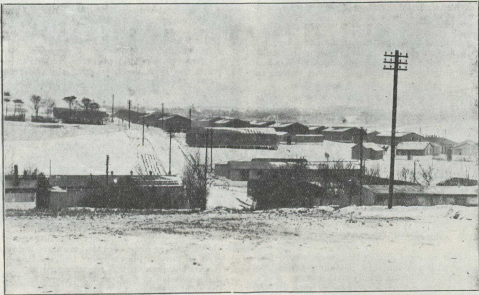
No. 3 Lines, looking East.
