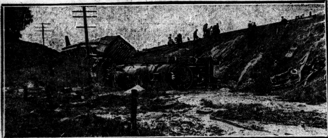
A heavy cloudburst in Indiana undermined part of a railroad track. When this long express train attempted to cross a filled-in valley, the cave-in and wreck occurred, killing the engineer.
