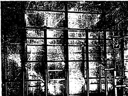
Fig. 4. WASHING DEVICE THROWING TWO SOLID SHEETS OF WATER AT RIGHT ANGLES WITH THE FLOW OF INCOMING AIR.
