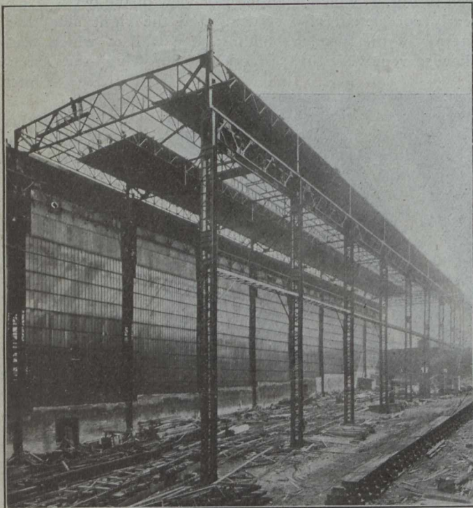
Fig. 2.—Erection of First Section of Berth. All the Glass and Sash in the Side of Adjoining Building was Later Removed
