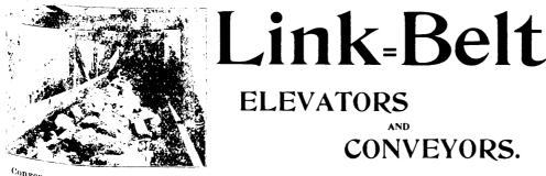
Conveyor 328 feet centers, handling 4 tons "run of mine" coal per minute.
