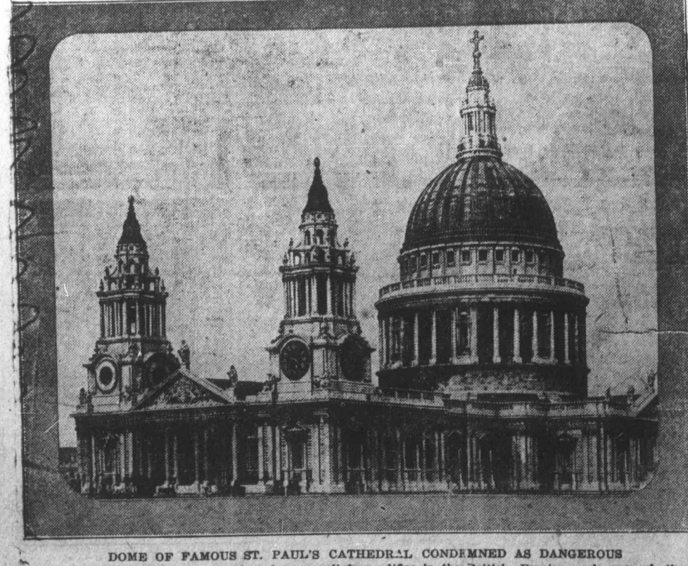
DOMES OF FAMOUS ST. PAUL'S CATHEDRAL, CONDEMNED AS DANGEROUS. A striking picture of the most famous religious edifice in the British Empire and one of the world's great Cathedrals, St. Paul's in London, England. The architecture of this building is the work of the noted Sir Christopher Wren. The hollow pillars supporting the dome must be replaced with new solid ones.
