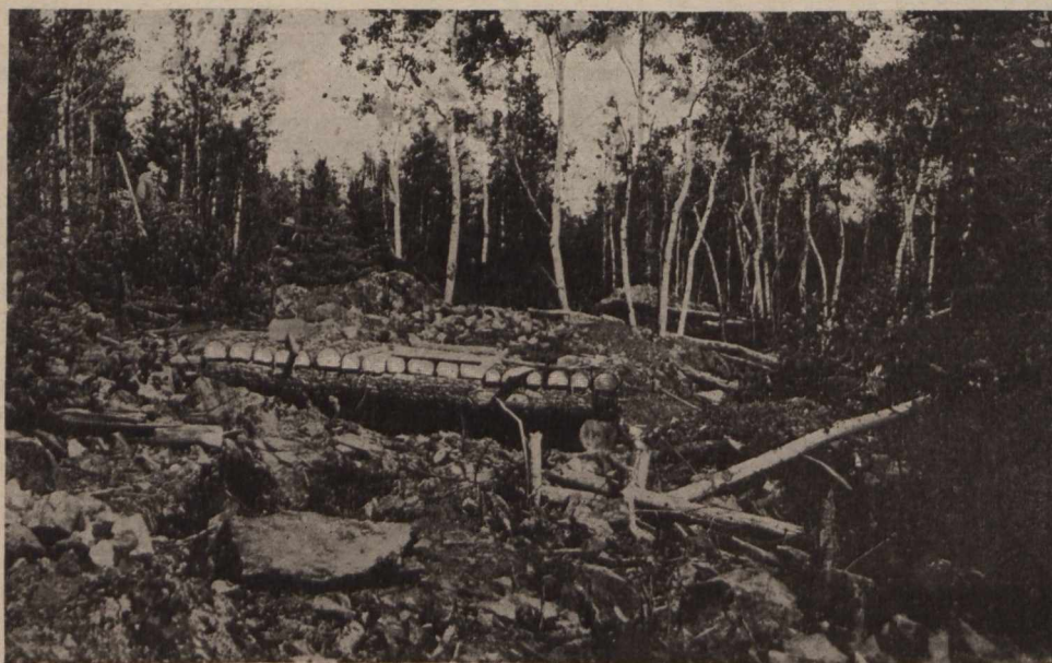
The Roofed-Over Pit sunk on the rich gold-shoot on the "Red Rose" at Copper Lake, Man., which first called attention to this district.
