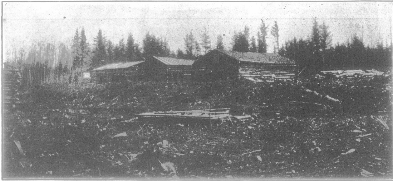
DINING HALL OF CONSTRUCTION CAMP, THREE MILES FROM END OF STEEL, IN JUNE, 1906.
