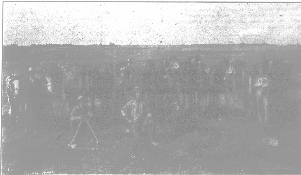
A ROAD CONSTRUCTION GANG, WARD 5, BIRTLE, MAN.
