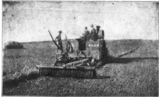
Showing the Centre Section of our Mulcher attached to an Engine Plow
