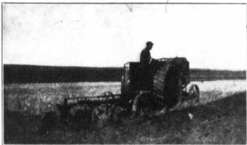
A Sawyer-Massey Kerosene Burning Tractor doing a fine job of plowing.
