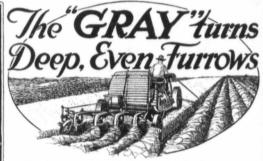
The advantage of the wide drive drum as used in Gray Tractor is greater traction surface and the elimination of soil packing, the weight being distributed over a large surface. Packers or disks attached to the side arms with a 26-ft. drag, will prepare 60 acres of seed bed in a ten-hour day.
