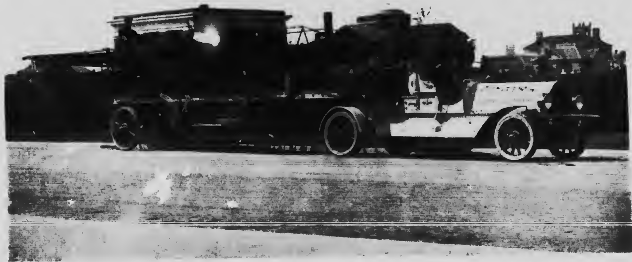
UP-TO-DATE MOTOR FIRE FIGHTING EQUIPMENT IS USED IN REGINA
