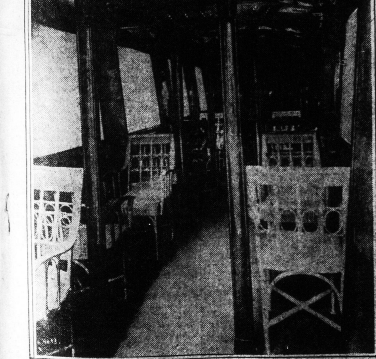
INTERIOR OF ONE OF THE CABINS OF THE ZEPPELIN AIRSHIP DEUTSCHLAND
