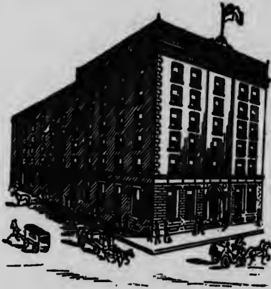
The Hudon and Orsali Building.
