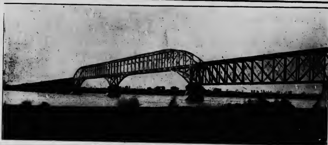
ST. LAWRENCE RIVER BRIDGE, C. P. RY., LACHINE, P. Q.—BUILT 1886
