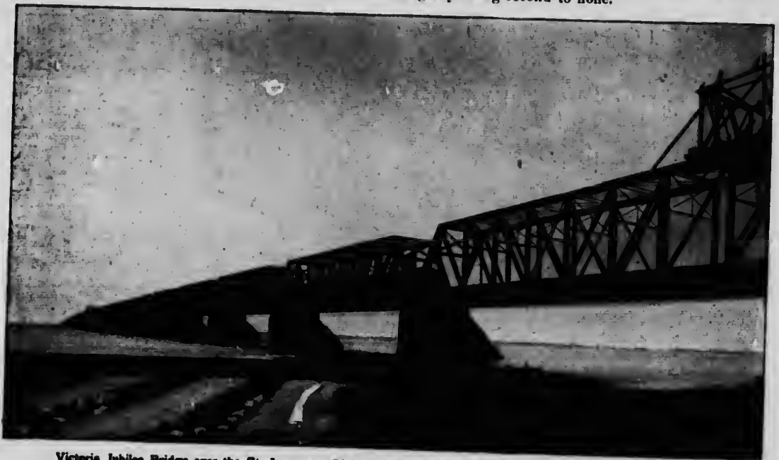
Victoria Jubilee Bridge over the St. Lawrence River, Montreal, said to be the longest Bridge on the Continent.
