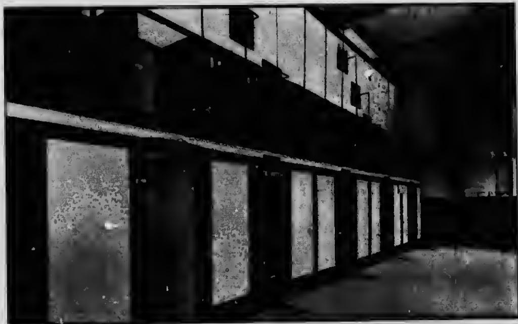
Concrete Compartments and Safety Gates on High Tension Side, also Electrolytic Arresters.
