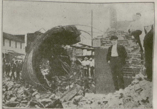
REINFORCED CONCRETE CHIMNEY BLOWN DOWN BY HIGH WIND.
