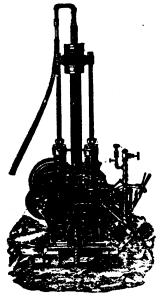
For prospecting Mineral Veins and Deposits, Boring Vertically, Horizontally or at any angle, to any desired depth, taking out a Cylindrical Section or Core the entire distance, showing exact character, and giving a perfect section of the strata penetrated. Also for Boring Artesian Wells perfectly straight, round and true.
