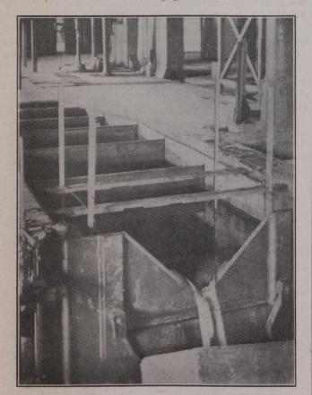
FIG. 2. Showing Method of Varying the Width and Depth of Channel of Approaches.
