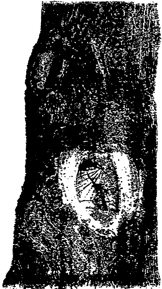
FIG. 223. Decay caused by the cutting of too large a limb. (By permission from U. S. Year Book of Agriculture, 1907.)
