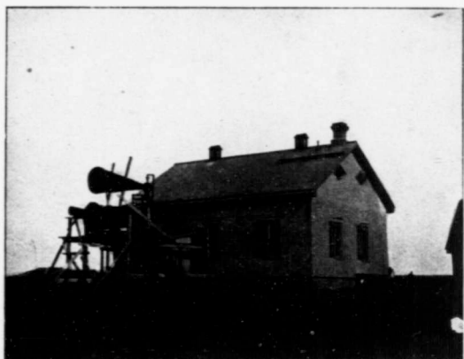
FATHER POINT (QUE.), FOG ALARM BUILDING—EXPERIMENTING WITH TRUMPETS
