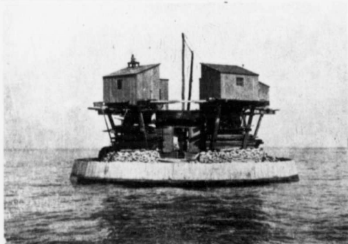
PELEE PASSAGE LIGHTHOUSE—FOUNDATION PIER 7
