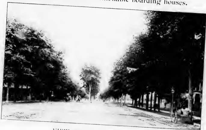
VIEW ON CIRCULAR STREET.
