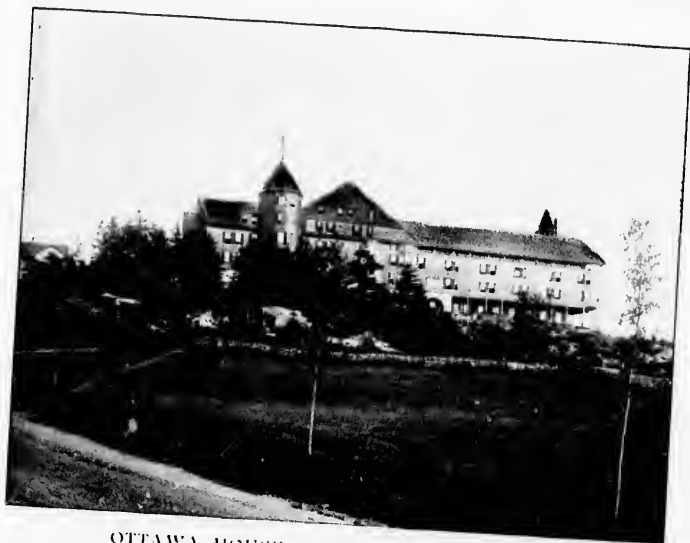
OTTAWA HOUSE, CUSHING'S ISLAND, ME.
