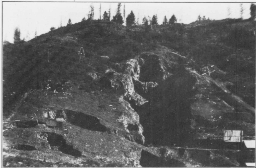
Ciel ouvert, Mine Granby, Phoenix, C.-A.
