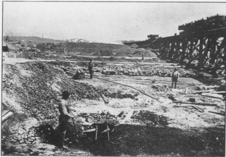
Terrains de grillage, smelter de la Canadian Copper Co., Copper Cliff (Ont.).
