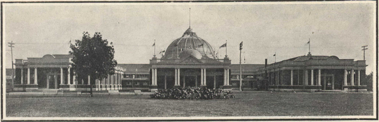
The New Agricultural Building.—A Rear View.
