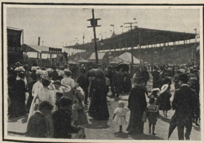
The new Grand Stand which seats 15,000 people. It is almost entirely of steel and cement.
