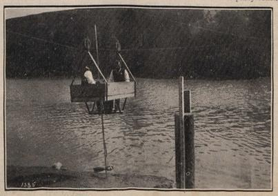
Cable Car and Gauge Height, Elbow River, Alta.
