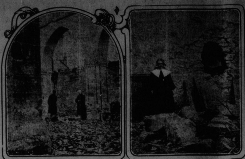
INTERIOR VIEW OF THE CHURCH AT LE MAUPLY SHOWING THE ALTAR. HOLE MADE BY BOMB IN CHURCH AT GIBEVELERS.
