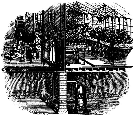
"Little Giant Heater" (Improved) installed to heat a Conservatory. This type of "Little Giant" will supply hot water for the bath, laundry and kitchen, as well as give the required radiation.
