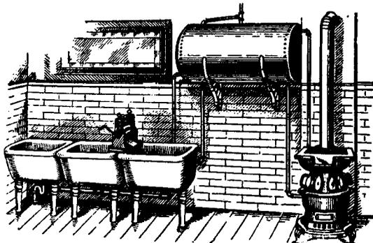
A Little Giant Laundry and Tank Heater is here installed in the cellar, with the hot water reservoir suspended from the ceiling over the stationary tubs. This arrangement saves space and removes the reservoir from the cold surroundings of the cellar floor.
