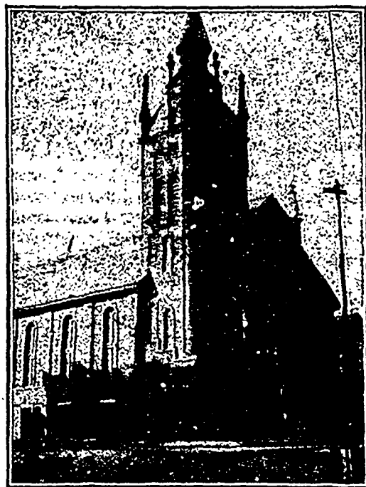
CENTRAL PRESBYTERIAN CHURCH, DETROIT, Headquarters for Canada and District of Columbia.
