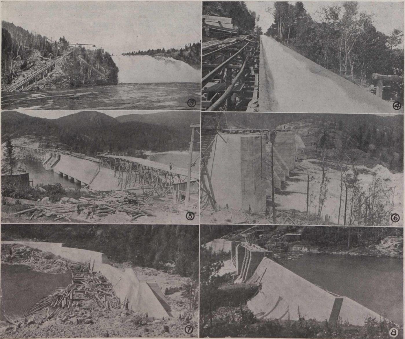
Fig. 3.—View of work from downstream side. Fig. 4.—A portion of the log slide showing uniformity of depth of water. Fig. 5.—Submerged intakes and sluice openings of south channel dam. Log slide intake in the right foreground. Fig. 6.—Showing clean discharge of piers. Fig. 7.—The north channel dam. Fig. 8.—South channel dam from island. The 200-ft. of 217 crest in foreground.
