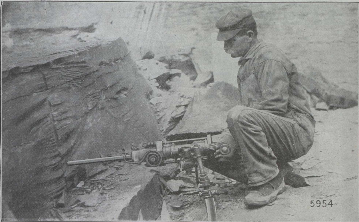
B.C. 430 HAMMER DRILL IN OPERATION
