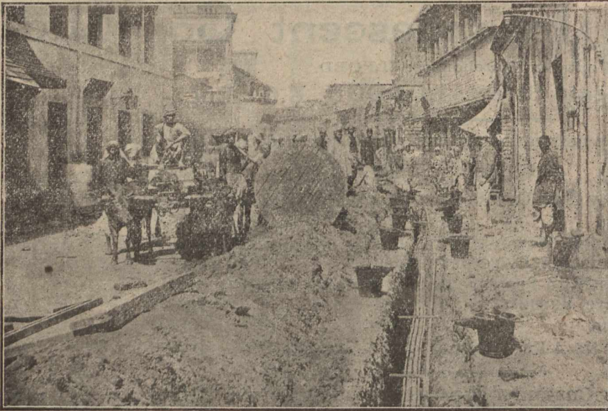
Laying Callender Mains at CALCUTTA.
