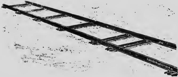
FIG. 122—Portable Tracks used on Peat Bogs.
