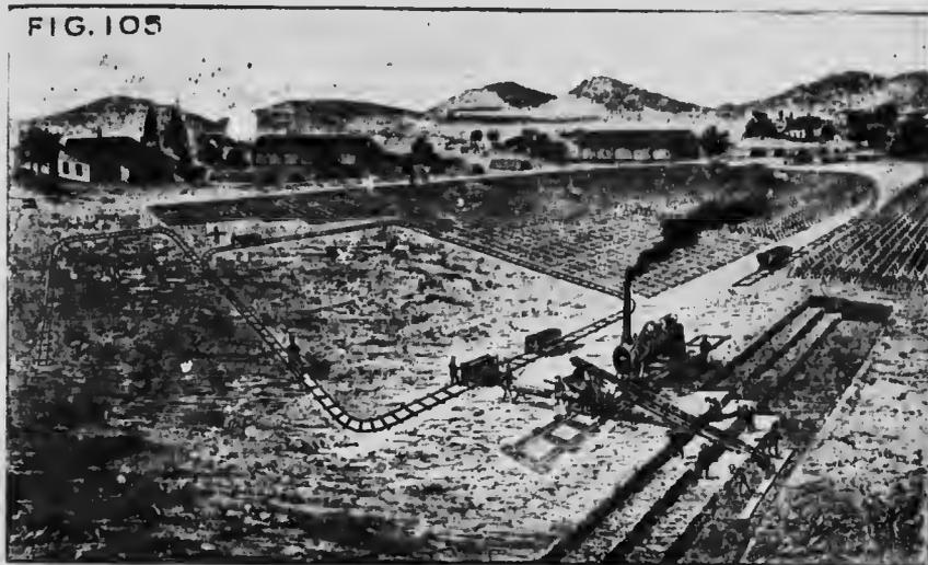
FIG. 105—General arrangements at a Dolberg Peat Plant with Peat Machine No. 1, h. or l. c. (in a drained bog).
