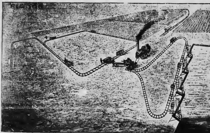
FIG. 106—General arrangements at a Dolberg Peat Plant with Peat Machine No. 1, b. and Cutting Machines (in a wet bog).
