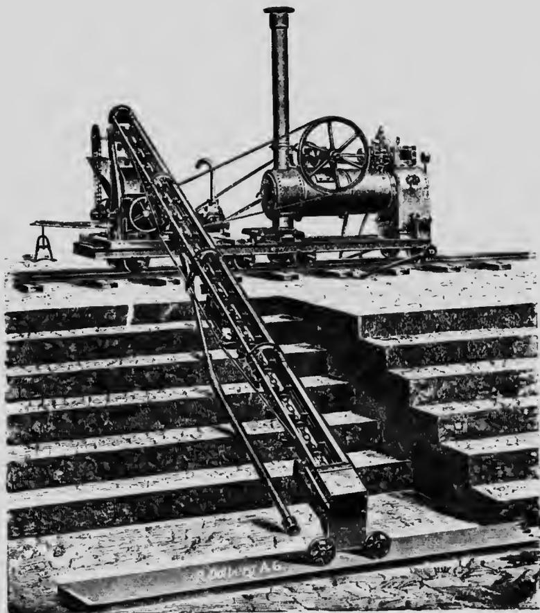
FIG. 68—R. Dolberg's Peat Plant with side elevator.
