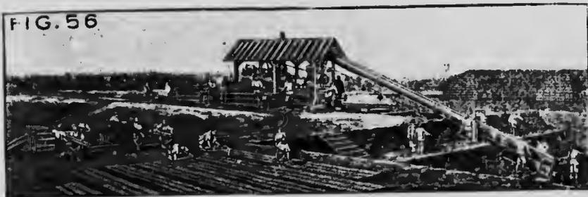
FIG. 56—Schlickeysen's Peat Machine with end elevator.
