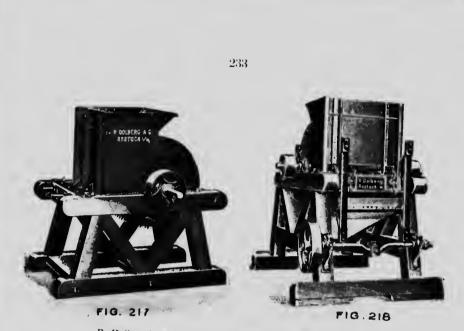
R. Dolberg's Moss Litter Disintegrator for Motor-power.
