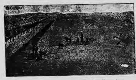
FIG. 99—General arrangements at a Dolberg Peat Plant with a one horse Peat Machine (in a wet bog).
