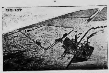
FIG. 107-General arrangements at a Dolberg Peat Plant with Peat Machine No. I. b. and Cutting Machine for Motor-power.
