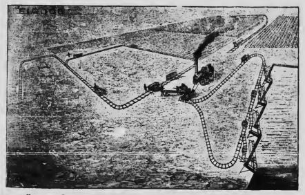
FIG. 106—General arrangements at a Dolberg Peal Plant with Peat Machine No. I. b. and Cutting Machines (in a wet bog).
