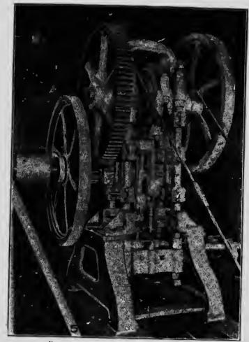
FIG. 165-The D., kson Peat Briquetting Press.
