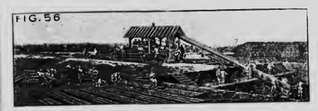
FIG. 56-Schlickeysen's Peat Machine with end elevator.
