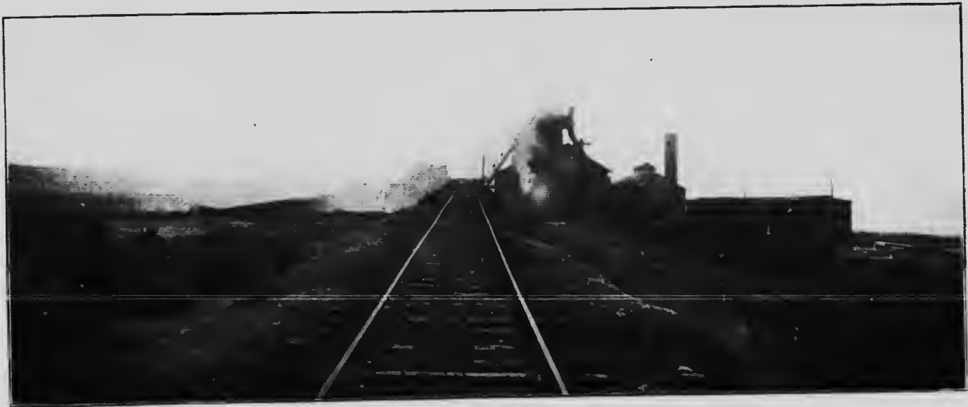
THE ATIKOKAN IRON CO.'S BLAST FURNACE, PORT ARTHUR
