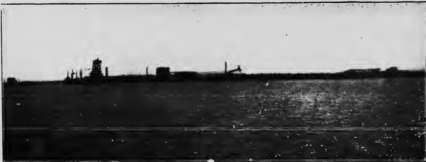
BIRD'S-EYE VIEW OF THE COAL DOCKS AT PORT ARTHUR
