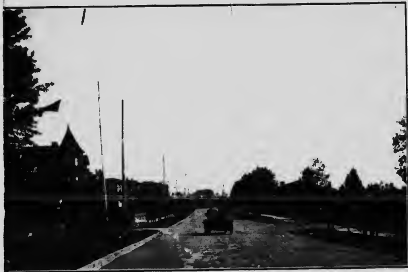
PORT ARTHUR'S MAIN STREETS, BOTH BUSINESS AND RESIDENTIAL, ARE PERMANENTLY PAVED
