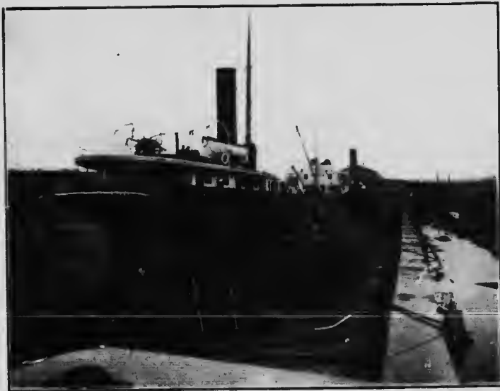
The Dry Dock of the Western Dry Dock and Ship-Building Company, 700 feet in length, 80 feet wide at the base and 100 feet wide at the crown.
